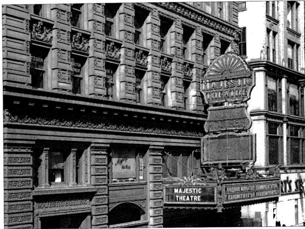
The Majestic marquee, circa 1930. Over time, the theater's marquee has undergone several changes. The original marquee, with the additions of lights, lower trim and an ornate blade, appears in this photograph.
